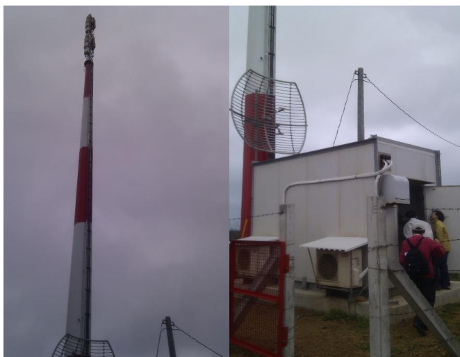
Fig. 1 Gap filler construction (a site in Peng Hu County)
